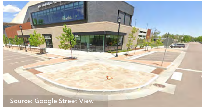
Source: Google Street View Curb extension reducing turning radius at Tejon and Dale streets.
