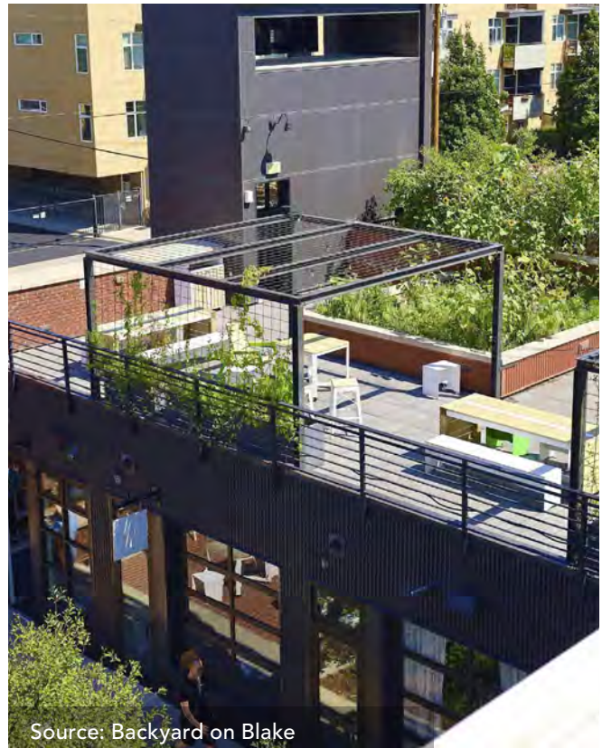
The Backyard on Blake courtyard and commercial spaces in Denver, CO, provide a publicly accessible rooftop available for everyone. It also hosts an urban garden and occasional events.
