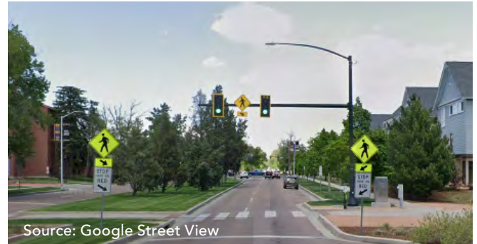
Source: Google Street View Pedestrian hybrid beacon across the northbound lanes of Nevada Avenue.
