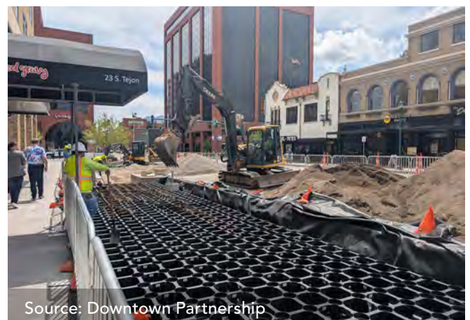
Soil cell installation along Tejon Street
