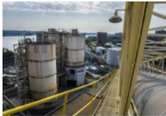
Potomac River Generating Station. Photo courtesy Hilco Redevelopment Partners
