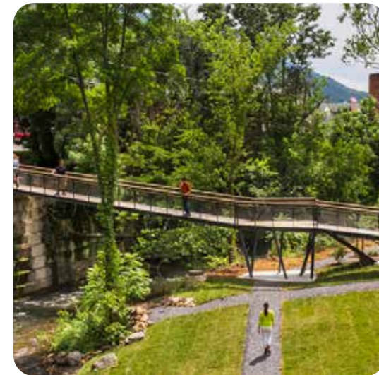
Signature pedestrian bridge
