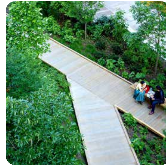
Water quality boardwalks
